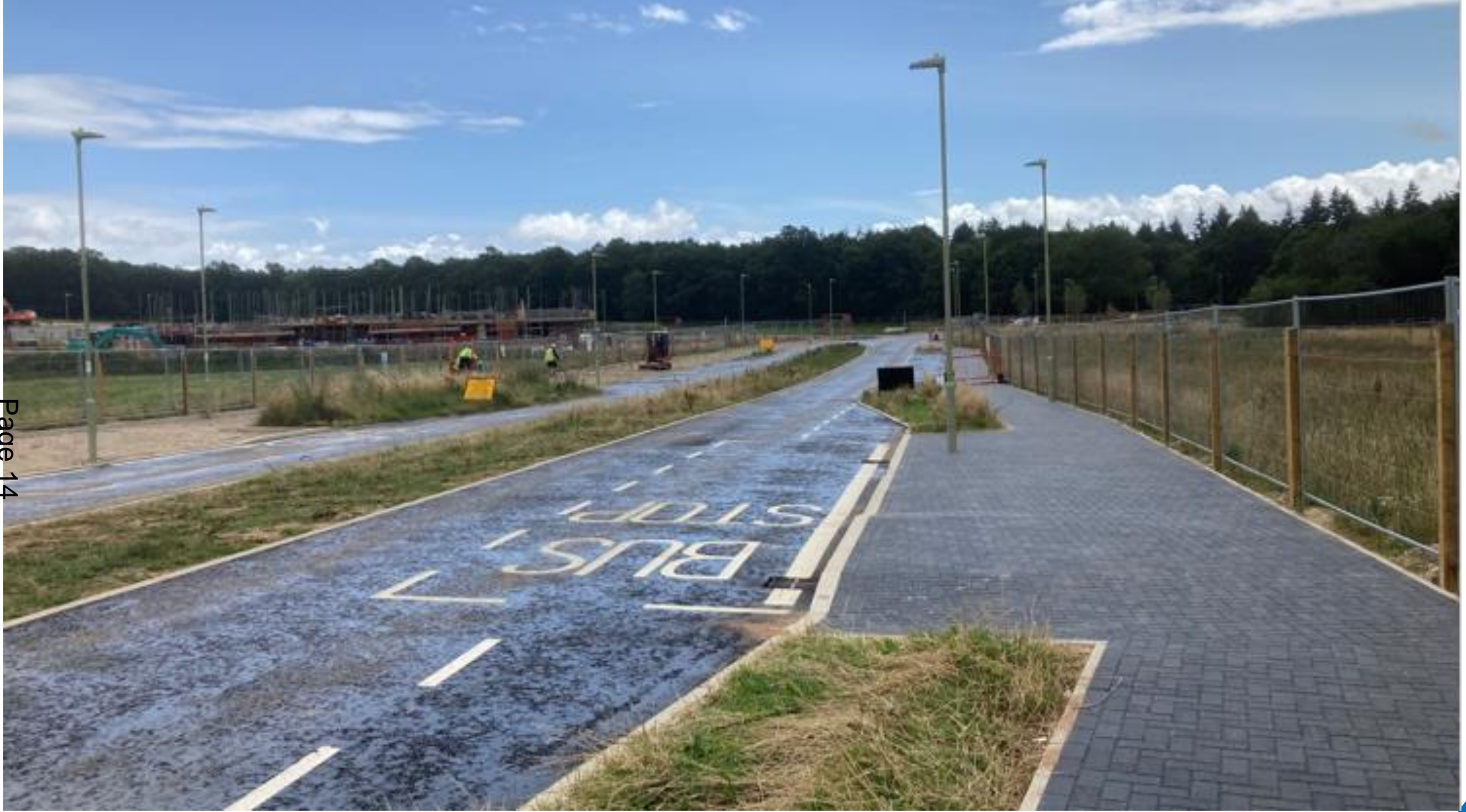
Phase 3 Whiteley Way South (Jan 2023)
