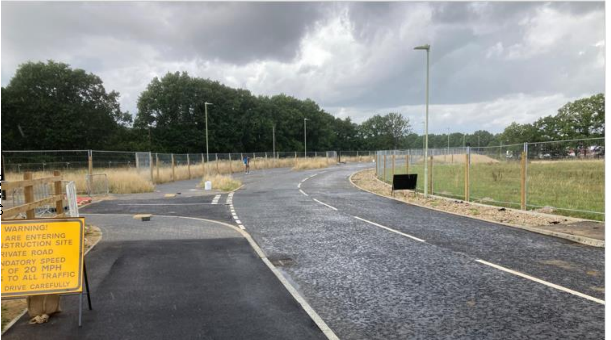
Phase 3 Curbridge Way (July 2023)
